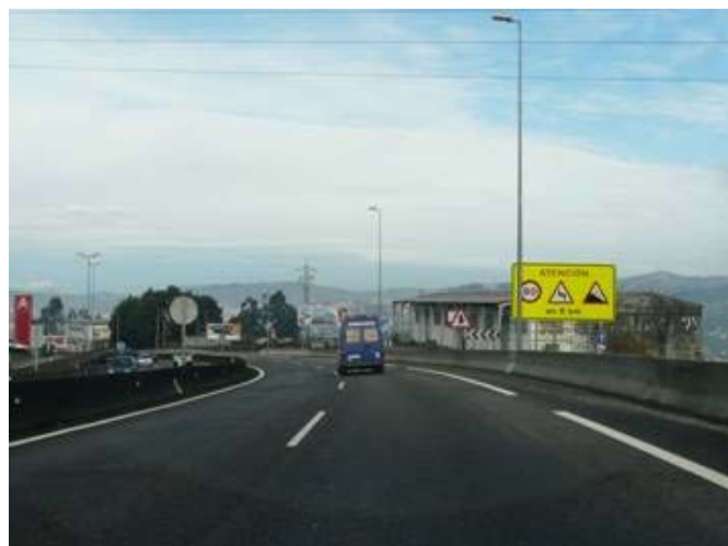
Figure 3 Sharp Bend in Spanish Test site.
