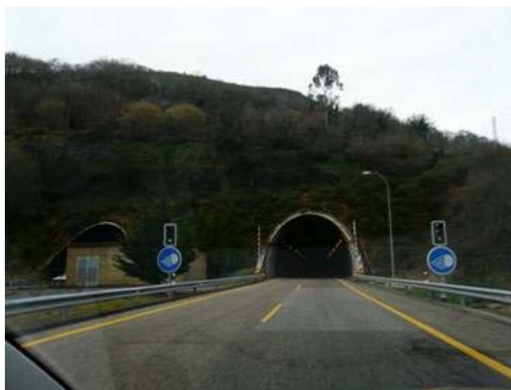
Figure 5 Tunnel in Spanish Test site
